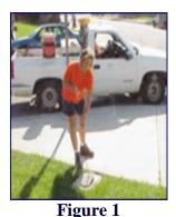
Your water meter is generally located near the curb in front of your home although in some areas it may be inside your home, usually in the basement. Outside meters are typically housed in a concrete box marked "water" (as shown in Figure 1) or in a meter pit with a cast iron lid. Carefully remove the lid by using a tool such as a large screwdriver or pliers and visually examine the area around the meter to make sure there are no harmful insects or other animals.
